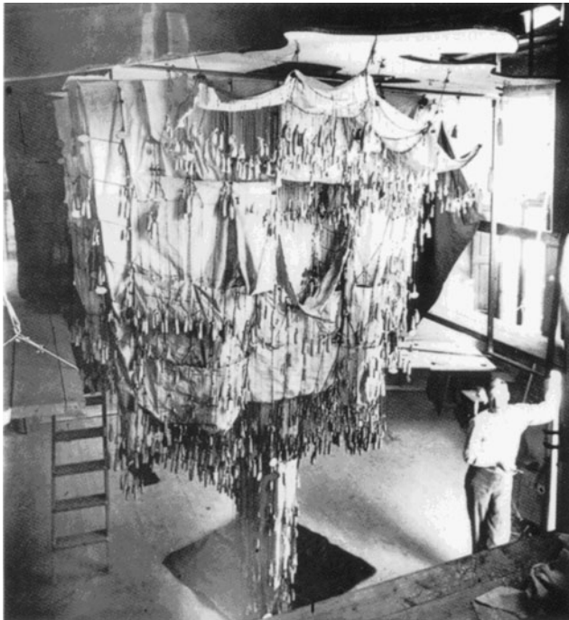
Fig. 10 Gaudi's hanging model used to design the church of Colònia Güell c. 1900 (Ràfols [118])
