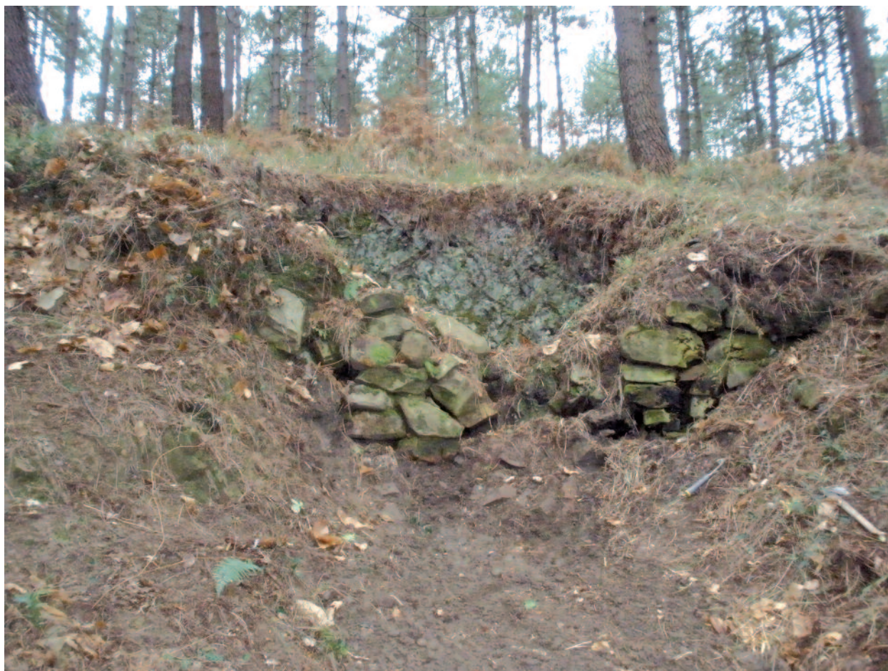
Figure 7. Front of the furnace of Erletxe in Galdakao, showing the sandstone wall that reinforces the structure.
