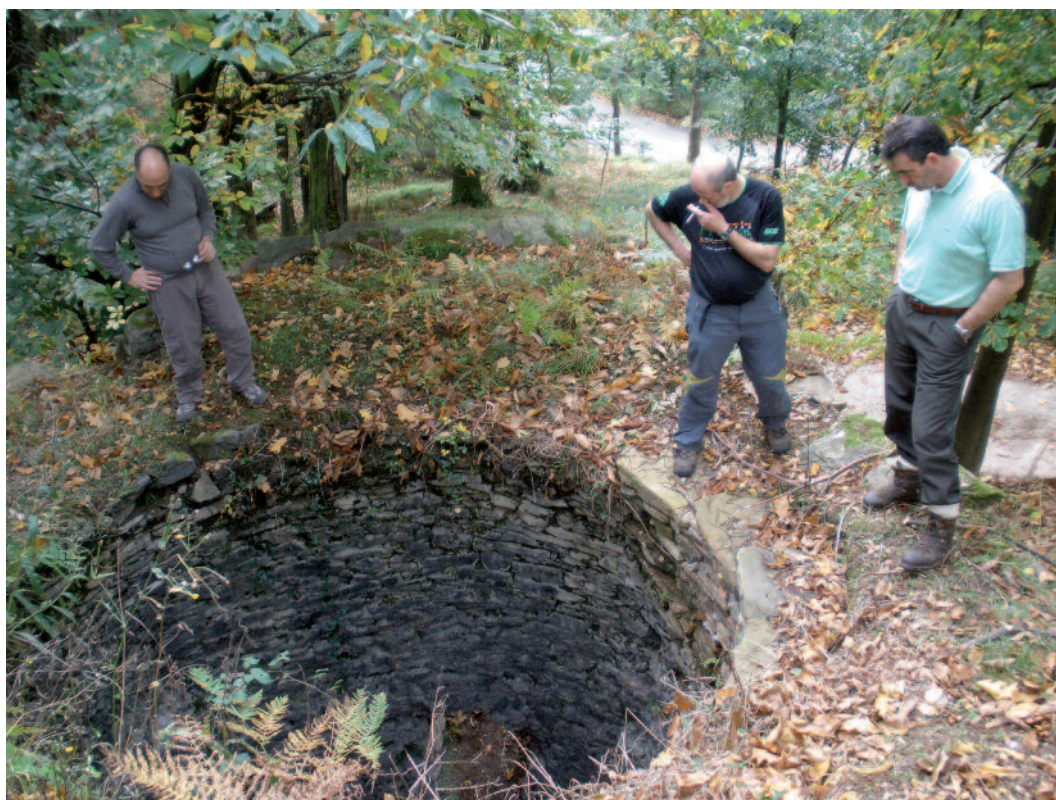
Figure 11. Inner view of a lime kiln (Leitza, Navarra), with the inner wall lined with sandstone and an approximate diameter of 3 m.
